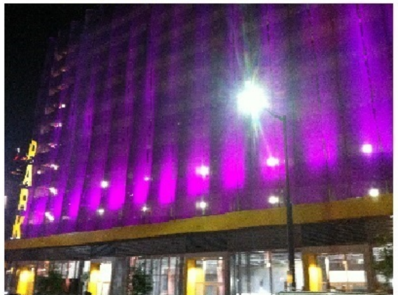
*ACTUAL PICTURE OF PARKING GARAGE*
